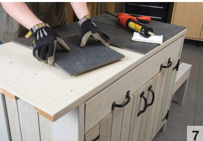
**Apply construction adhesive to the back of each tile and place the tile on the backer board, leaving roughly even spaces from the edge of the backer board and between the tiles.**
