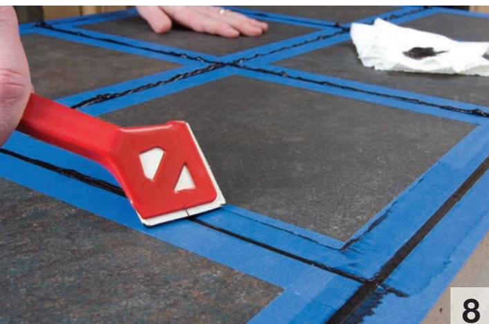
**Fill the gaps between the tiles and around the perimeter with silicone caulk. Screed off the excess caulk with a caulking-smoothing tool or plastic putty knife.**
