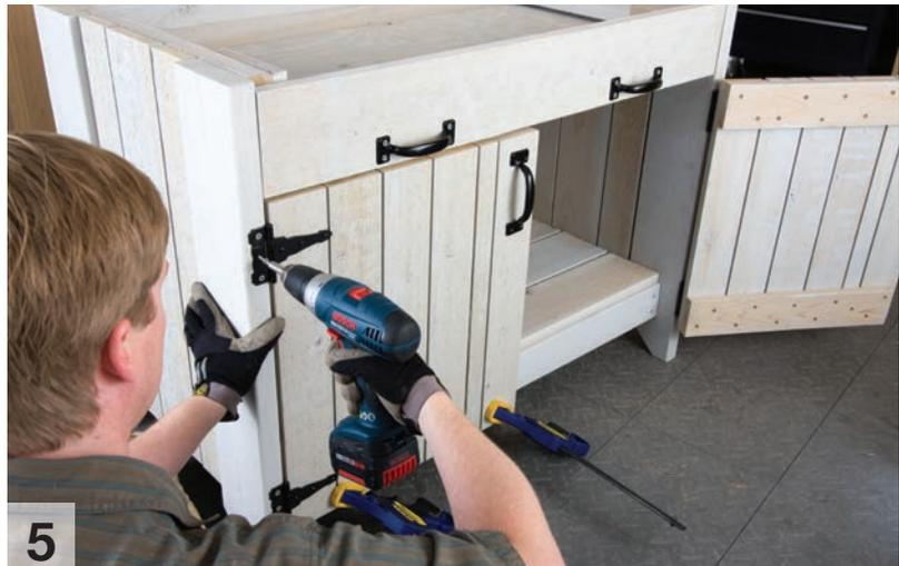
**5** Position the hinges so that the bottom/top edge of the vertical plate is 1 in. from the bottom/top edge of the doors.
