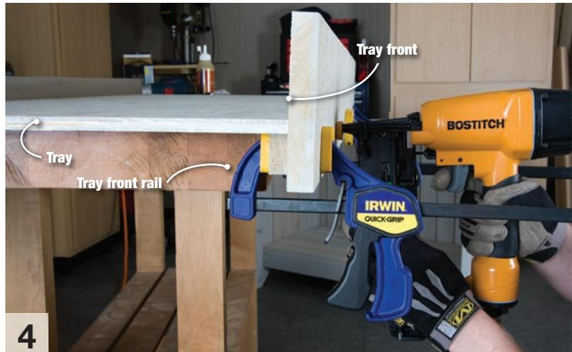
**4** Attach the tray front to the tray front rail with glue and finish nails. Then attach the handles with 1-5/8-in. screws.
